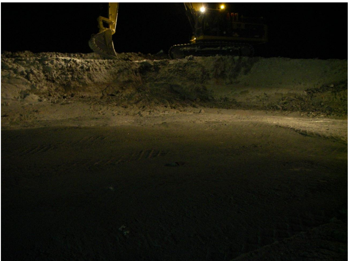
Photo 10: The CAT 345 excavator equipped with tiger teeth is removing the 5/8 crush in the south-west corner of the key-trench.
