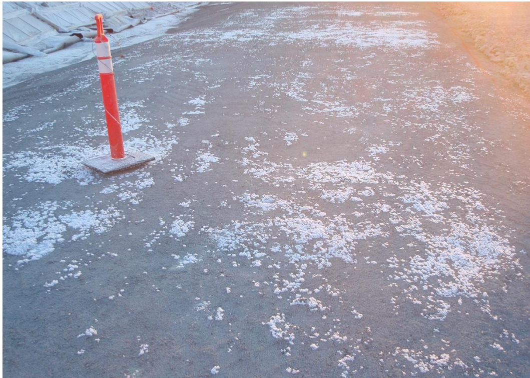
Photo 4: Last day's placement. Surface moisture has crystalized after placement.
