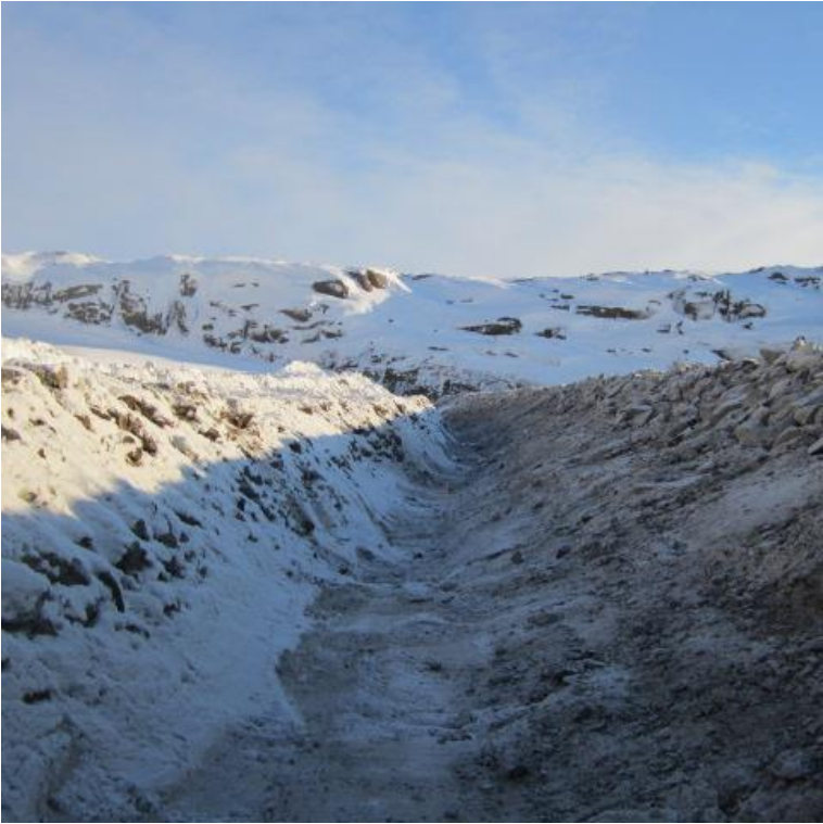
Photo 7: Photo looking down the diversion berm key-trench.
