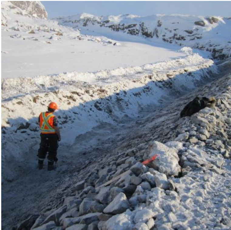
Photo 6: Doris North Diversion Berm looking east toward the east tie-in. Tundra and ROQ has been sloped. Bottom of the key-trench is free of excessive debris.
