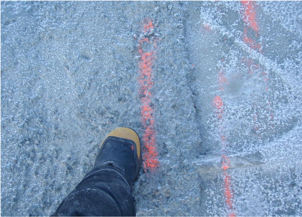
Photo 5: Small amounts of 5/8 crush imbedded near exposed liner.
